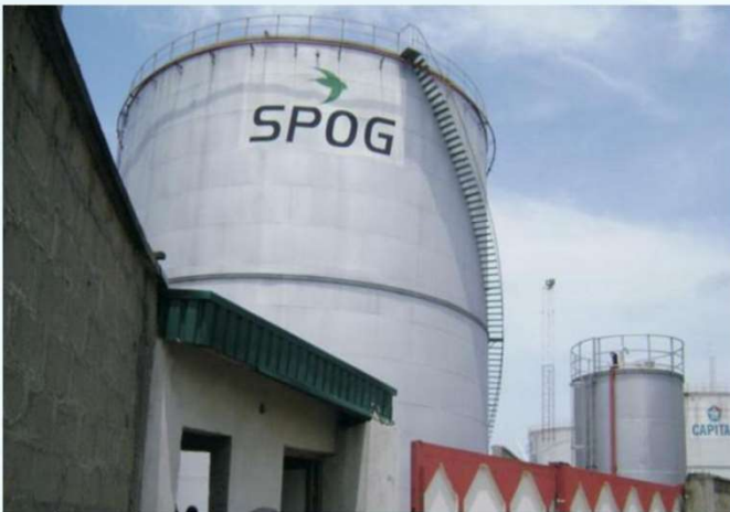
SPOG Petroleum Products Storage Tanks
