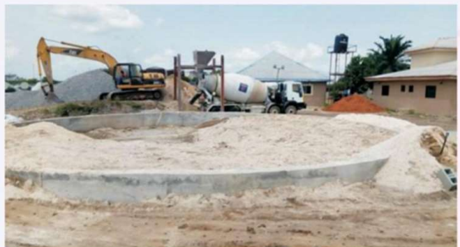
Construction of Tank Foundation
