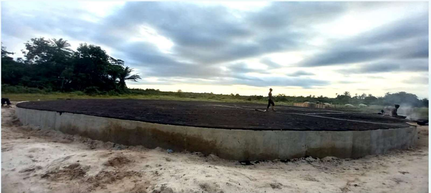
Completed Dwell Petroleum Tank Foundation
