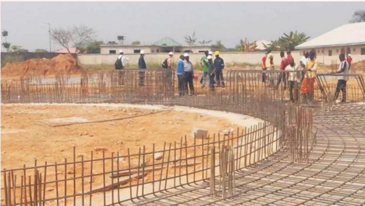
Civil Construction work of LPG Cylindrical Tank Foundation
