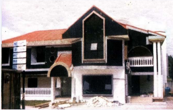
Residential Palace construction, Umuahia
