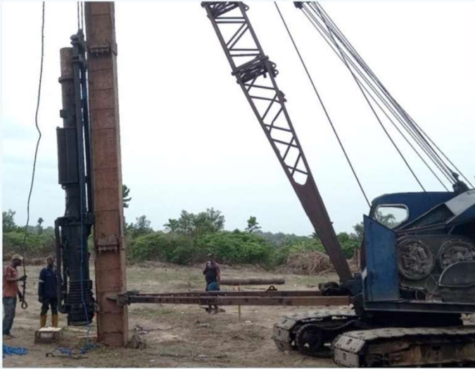
Vibro Stone Column (Soil Improvement)
