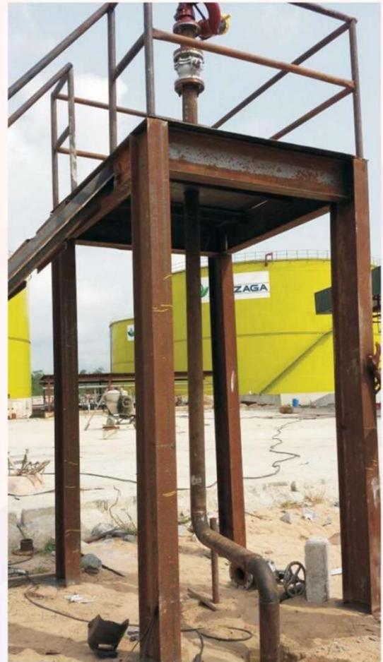
Fire Monitor Installation
