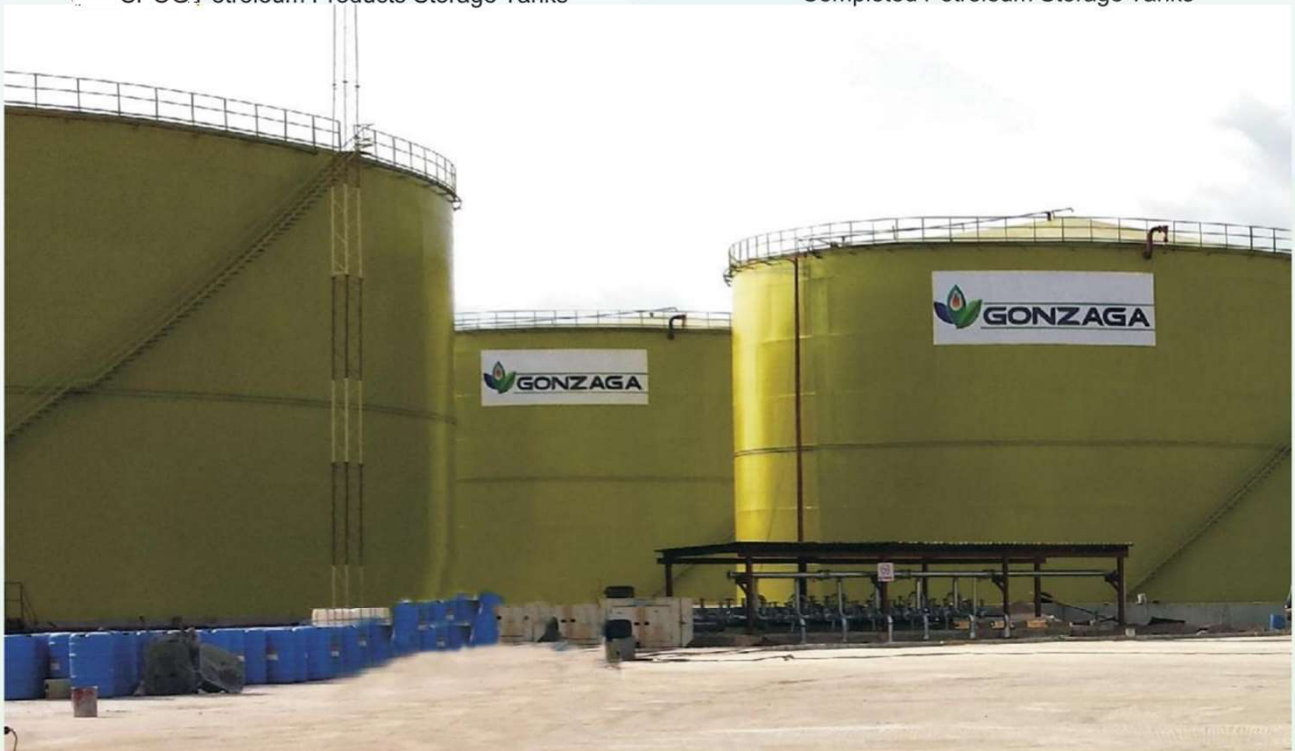
Completed Gonzaga Storage Tanks
