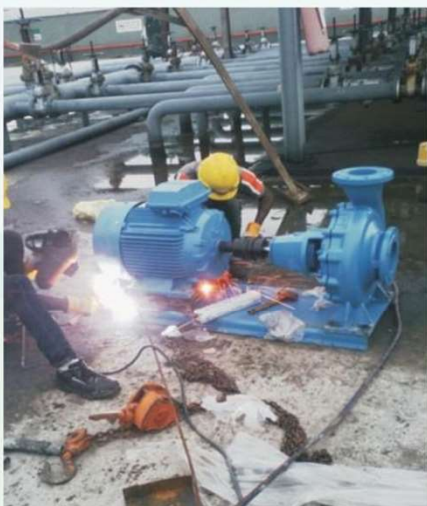
Installation of Pumps
