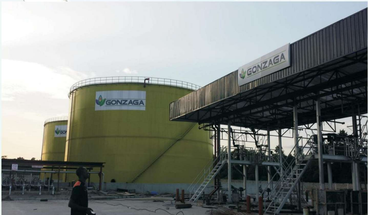
Gonzaga Tanks & Gantry
