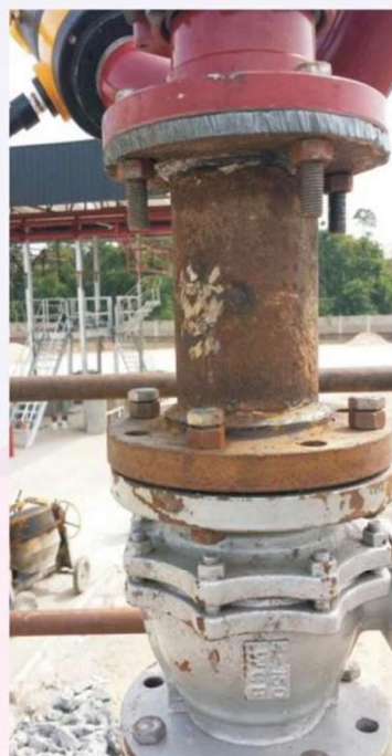
Fire Monitor Flange Construction
