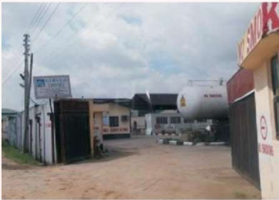
Allied LPG Plant
