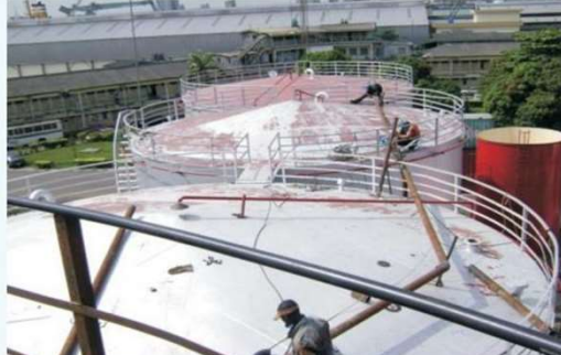
SPOG Petroleum Products Storage Tanks Reconstruction
