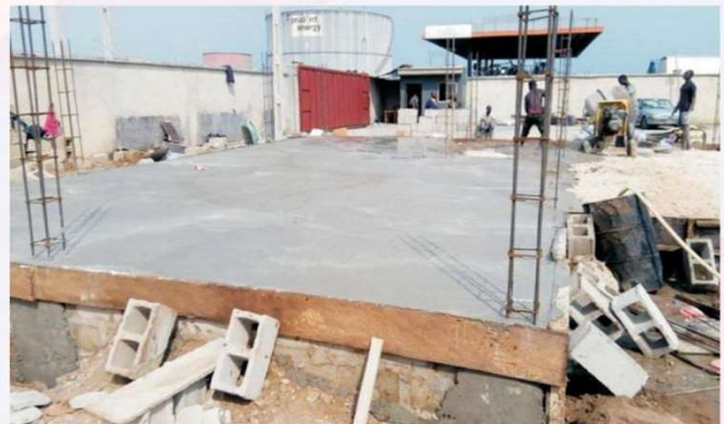
Petroleum Storage Tank Farm building Construction
