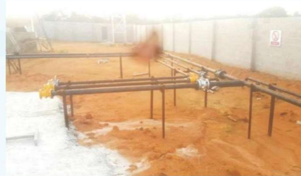
Abegas Port- Harcourt Pipeline works
