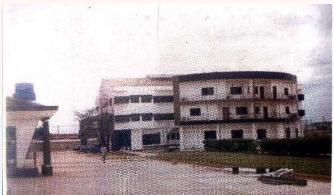
Construction of Damgrate Hotels, Umuahia
