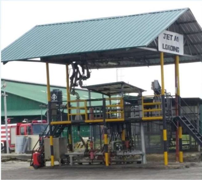
Renovation of loading gantry
