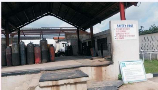
Allied LPG Plant Filling Bay
