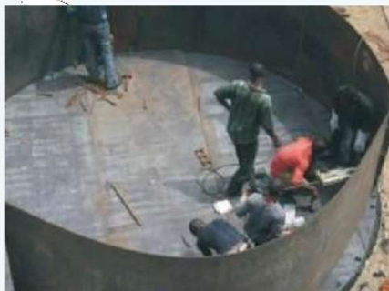
Construction of Tank base
