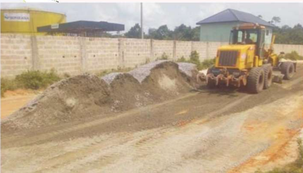
Road Construction to Gonzaga tank Farm
