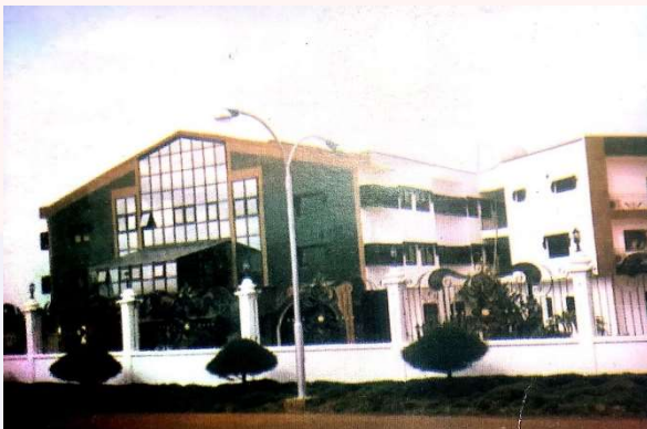
Construction of Damgrate Hotels, Umuahia
