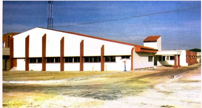
Construction of the Lekki British School, Lekki
