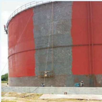
Painting of Tanks
