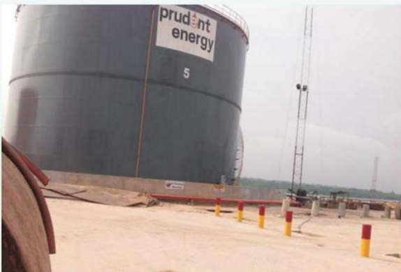
Prudent Energy Services Water Tank
