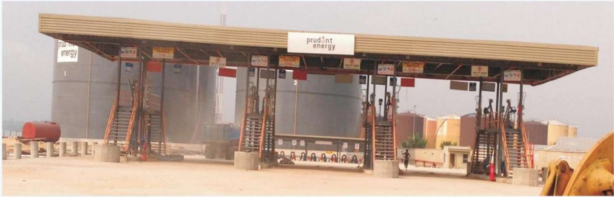
Prudent Energy Services Gantry
