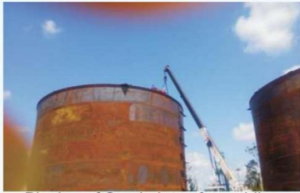
Placing of Steel plates for welding
