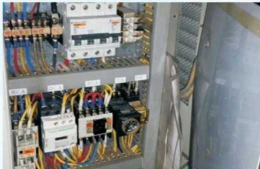
Electrical Installation at Gonzaga Tank Farm
